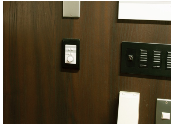
The MA2120 amplifier housed in the lower section of the counter (left) and the digital control panel DCP1V4S-US mounted on the wall.
