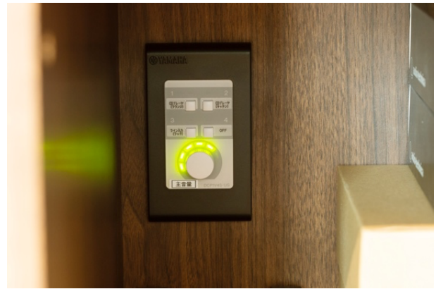
The AMX touch panel provides integrated control over video, audio, and BGM (left). A DCP1V4S-US digital control panel is also located inside the shelf to the right of the rack.
