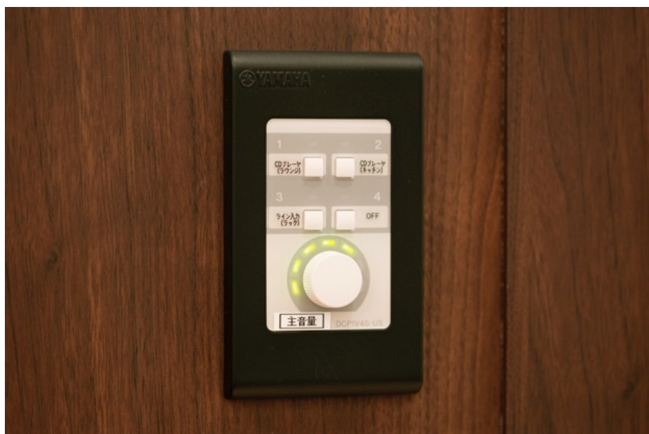
Wald Tür is equipped with three DCP1V4S-US digital control panels.
