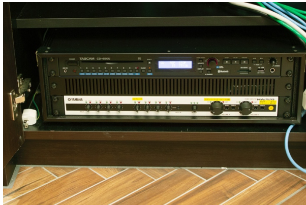
The MA2120 amplifier housed in the lower section of the counter (left) and the digital control panel DCP1V4S-US mounted on the wall.
