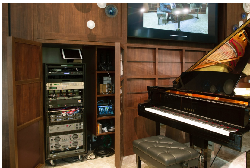
The audio equipment rack inside the front lobby wall cabinet.
