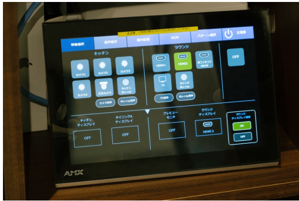
The AMX touch panel provides integrated control over video, audio, and BGM (left). A DCP1V4S-US digital control panel is also located inside the shelf to the right of the rack.
